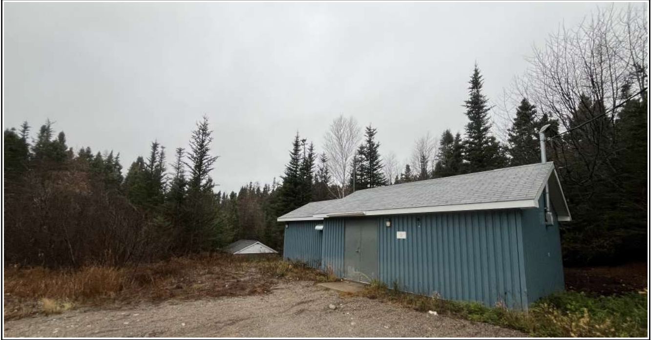
Illustration 16: Water Supply Pump House
